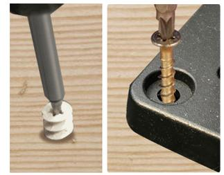
Insert the wall plugs into the drilled hole. Replace the bollard body lining up the 4 x holes at the base. Secure in place with 8mm screws.
